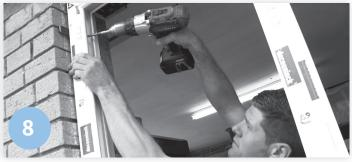
Output the second se is important to use plastic packers between the frame and the building at all fixings points to ensure that the frame is not distorted when tightening the screws.
