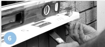
S Offer up the new frame and cill into the opening, using plastic packers ensure the frame is level and plumb whilst making sure that you maintain an equal expansion gap around the frame.
