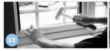
Now refit the beads in the same position as you removed them, start with the smallest lengths first before inserting the longer lengths. Use a rubber mallet/hammer to help tap the beads into position, focus on the edge where the bead meets the frame.
