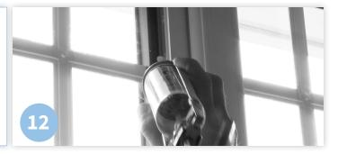
Once you are happy with the position of the glass packers and the glass sits square in the frame, test to make sure the sashes open and close correctly. Then, apply silicone either side of the packers to help keep them in place.
