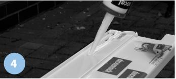
S Carefully silicone along the cill up-stand and at both ends, this is to prevent water and air leaks occurring between the cill, frame and surroundings.
