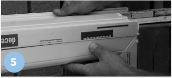
S Turn the frame over and secure the cill to the frame using the appropriate PVC screws. Fit the window handles.
