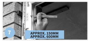
The frame is ready to be secured in place, fixings should be located  $\mathbf{G}$ approximately 150 in from each corner and then spaced at 600mm intervals, do not fix within 150mm of any mullions or transoms. Ideally you should use at least 2 fixings per side.
