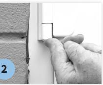
Once the centre hinge has been adjusted, open and close the door to make sure the lock is engaging. Once you are happy, replace the bottom cover cap.
