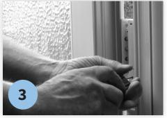
Once the vertical and lateral adjustments have been made to the hinges, you need to open the door and tighten up two locking screws top and bottom of each hinge. This allows you to fix the changes you have made.
